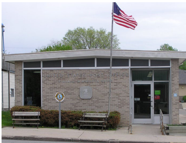
Pictured Above: Kimball Post Office
